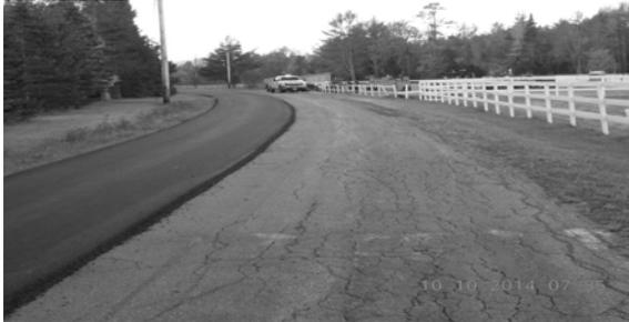
Cracked and broken pavement was ground up on Talbert Hill and Codfish Hill and prepared for paving in 2015.
