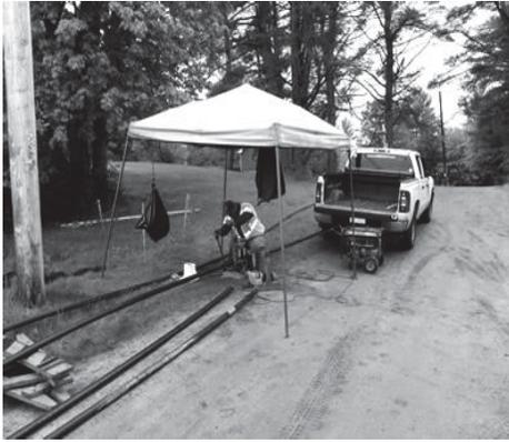
year old badly corroded 1 ½” galvanized pipe with a brand new 2” HDPE and installed a new 2” automatic blow off hydrant at the end of the line.
