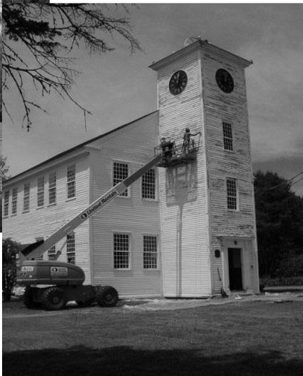
down through the clock works area of the tower, replaced the railings, replaced the roof under the bell and repainted the tower. The work was completed by Harvest Construction of Hartford, Vermont. The total cost was \$73,200. The Town paid
