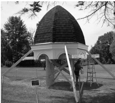
replaced the roof on the cupola, replaced beams
